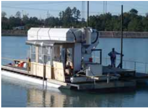
Barge-mounted unit applies bentonite materials clay to seal a leaking reservoir.
