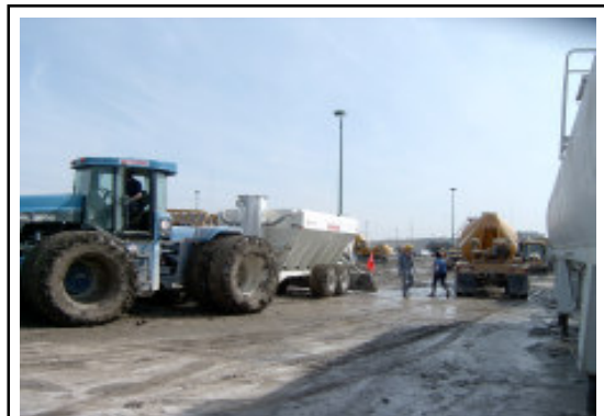
Transfer 1 ton of portland cement per minute from the tanker
